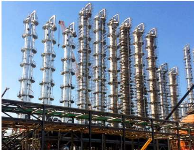
TBEA Polysilicon project
