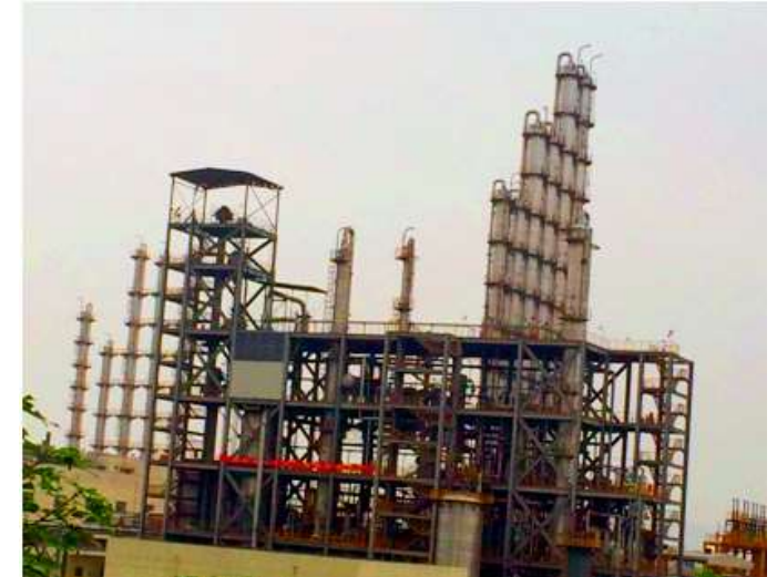
Yichang CSG Polysilicon Project
